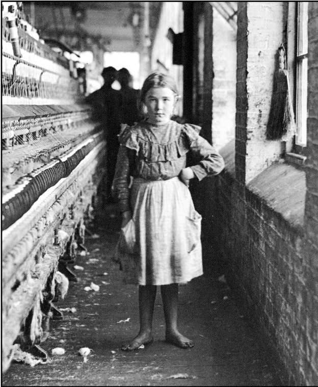
Source: Lewis Hine photograph
